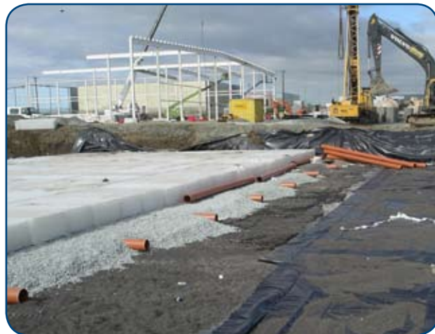
Stormcell ® Attenuation Tank under construction
