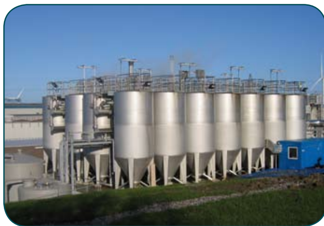
DynaSand® Filters continuously providing high quality process water to a box board manufacturing plant.
