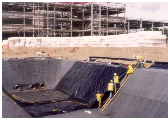
Stormcell® awaiting installation on site at Greenford Park.
