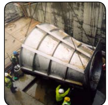
Installation of the Hydro-Brake® Flow Control
