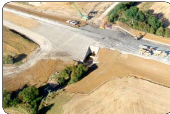
Aerial view of the dam during construction.
