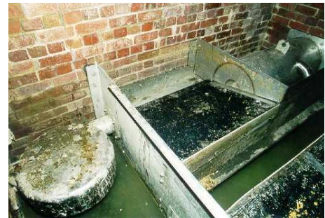
The Hydro-Jet™ Screen at Helmsley, following operation during a storm.
