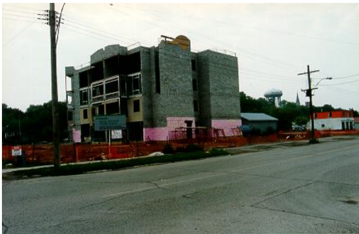
40-Unit Non-profit Housing Complex
