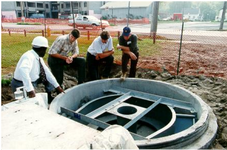
8.0 Ft. (2.4 m) diameter Downstream Defender
