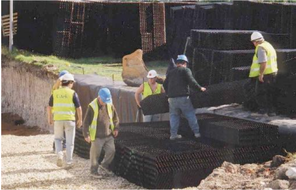
Figure 8: Typical Installation of Stormcell® Blocks
