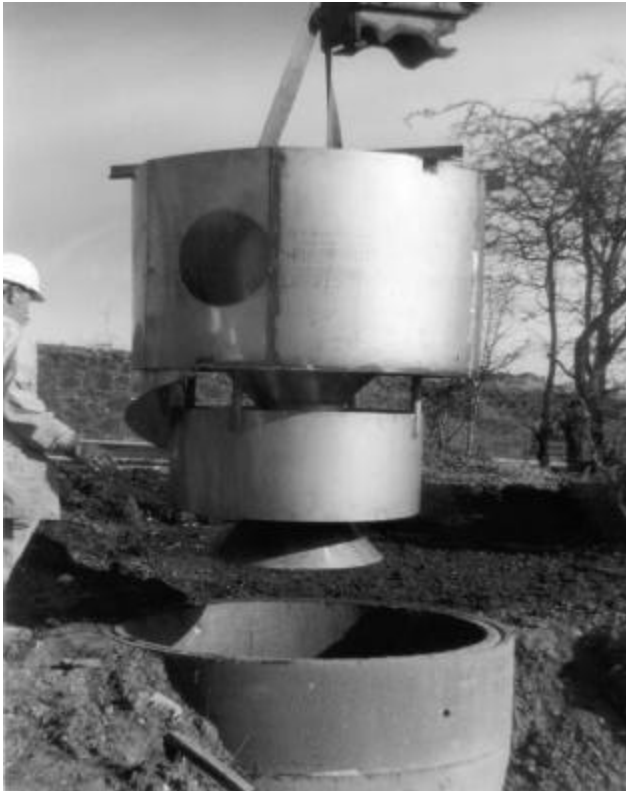
Figure 9 Installation of a Downstream Defender™
