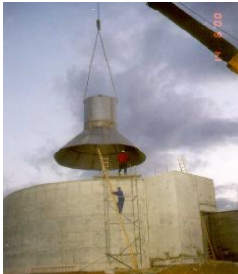
Figure 9 Internal Components Being Lowered into a 16m Diameter Swirl-Flo® HDVS
