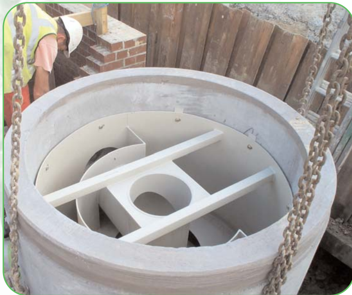
The 1200 mm Downstream Defender® During Installation
