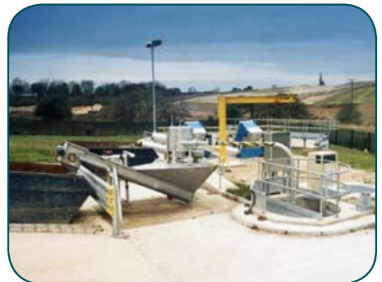
In Situ Grit King® Separator with Grit-Cleanse™
