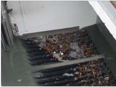
The Hydro-Jet Screen removes pollutant containing debris and circulates it back to the treatment plant.
