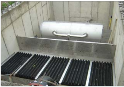
The satellite treatment system includes a Hydro-Jet Screen (pictured) and a Reg-U-Flo Vortex Valve flow control.
