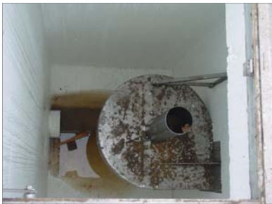
The Reg-U-Flo Vortex Valve returns the collected screenings flow to the wastewater treatment plant.
