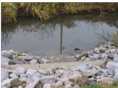
The screened effluent is discharged to nearby Raccoon Creek free of floatable debris.
