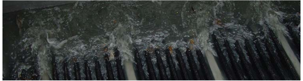
An integral airbrake siphon discharges screened water and provides the hydraulics for a self-backwashing mechanism that cleans the screen.
