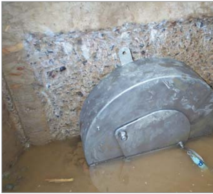
The Reg-U-Flo Vortex Valve supplied by Hydro International was chosen to serve as the basis for the inlet control system.
