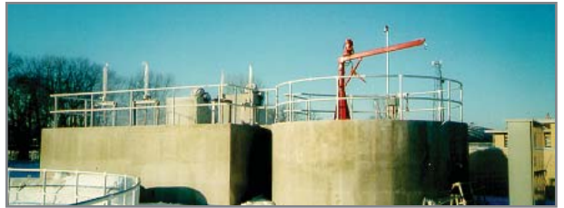
In situ units are designed for small or large applications ranging in size from 6 ft. in diameter to 40 ft. in diameter.
