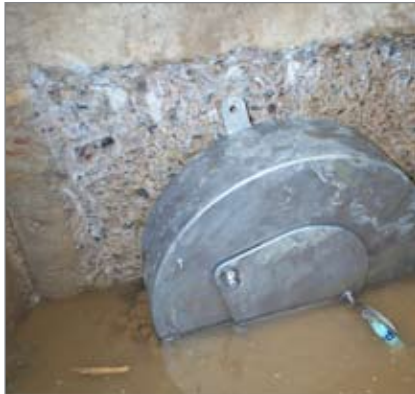
The Reg-U-Flo Vortex Valve supplied by Hydro International was chosen to serve as the basis for the inlet control system.
