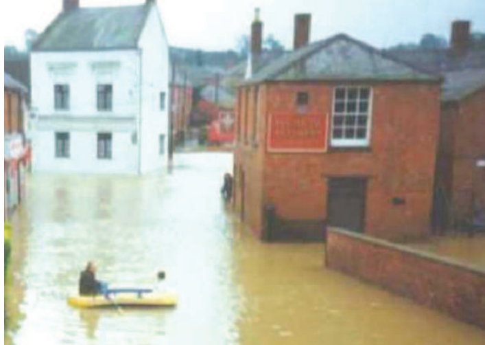
Flooding in the villages around Weedon disrupted 45 business and residential properties
