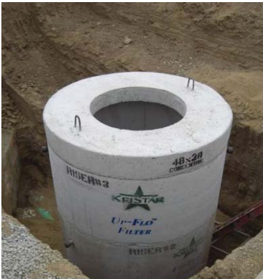
The Up-Flo Filter has a higher flow through capacity than traditional sand filters, making it a smaller and more economical alternative for stormwater treatment.
