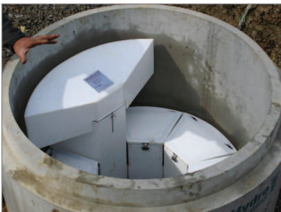
The Up-Flo Filter has a higher flow through capacity than traditional sand filters, making it a smaller and more economical alternative for stormwater treatment.
